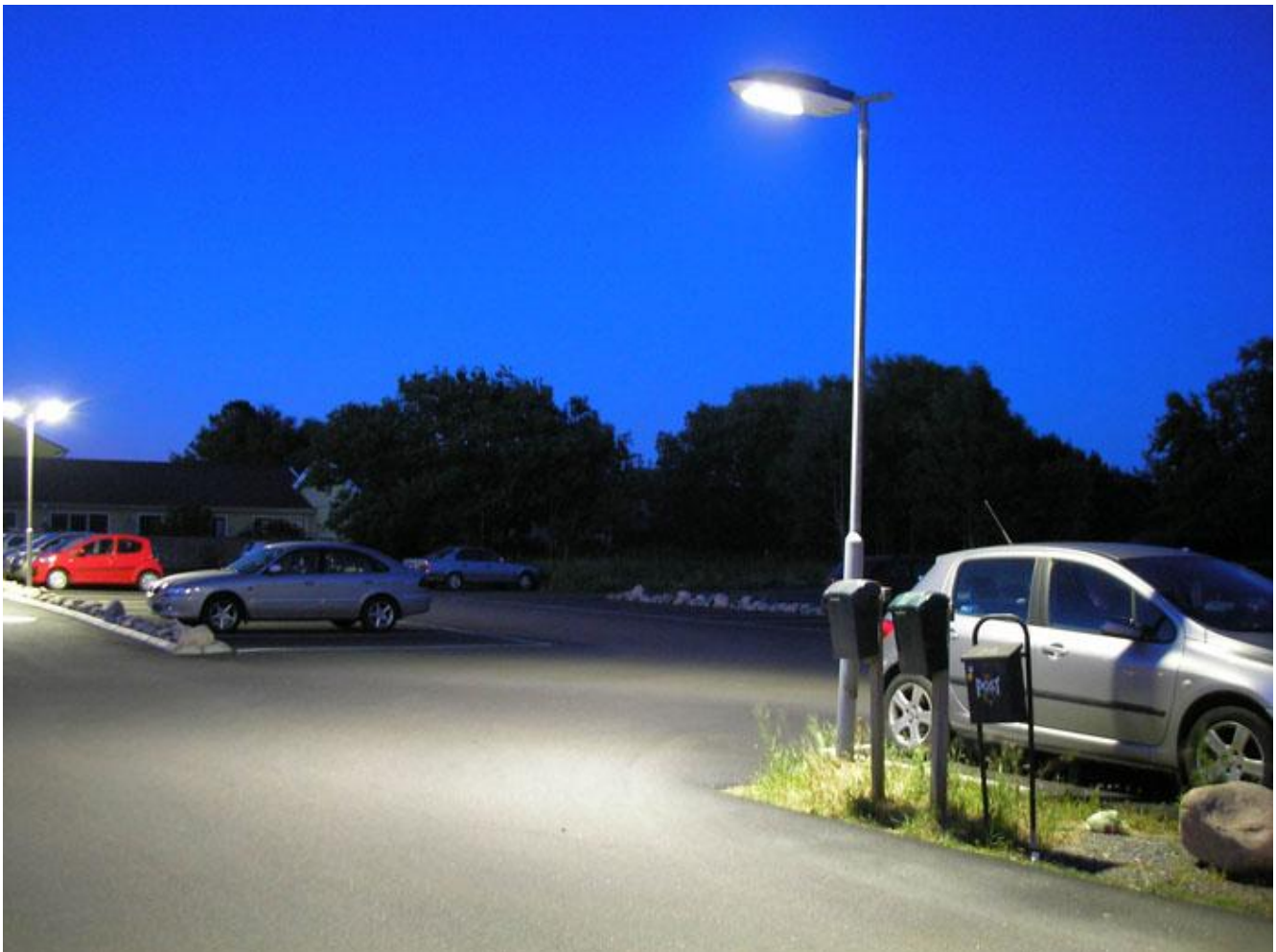
Figure 8: Parking lot Safety Lighting/LED technology
